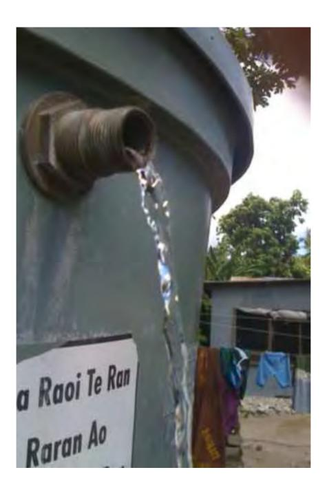
Above ground leak. The householder attempted to repair the leak at the connection by taping around the leaking fitting.
