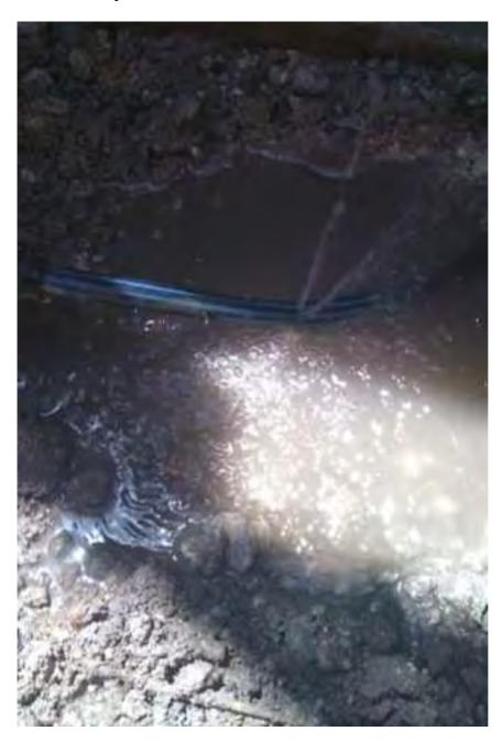
Leak found on 50 mm pipe with the aid of gas detector. Leak was caused by 2 cuts from a shovel
