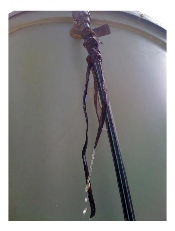
The largest underground leak detected and located. The actual leak had not been uncovered. This was aprox 25 cm below surface, and no moisture was visible on the ground. The leak was caused by some digging by the householder and hitting the pipe, probably with a shovel point. (See following photo)
