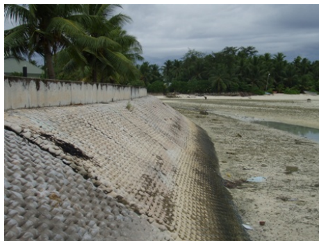
Revetment (sloping) seawall
