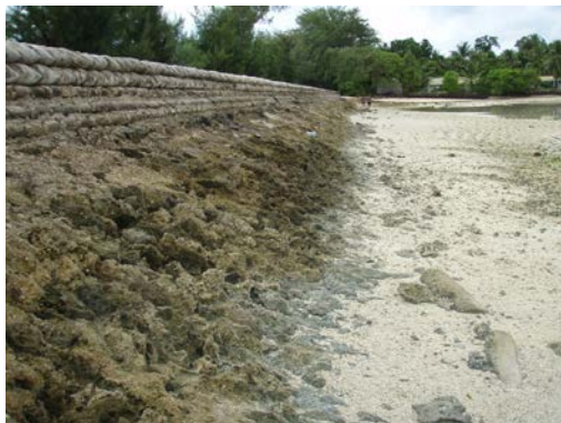
Rocks (1 layer, impermeable core)
