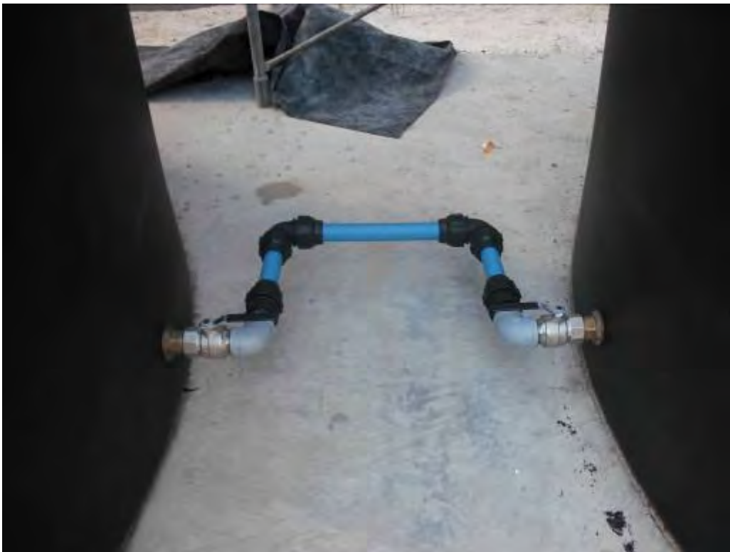
A1.3.2 Good tank connection, 50mm pipe with ball valves to isolate tanks
