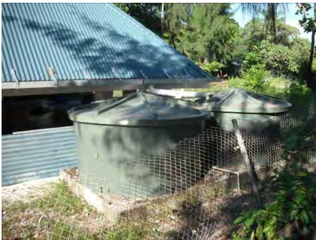
A1.3.6 Squat polytanks utilised where maneaba roof eaves are low.
