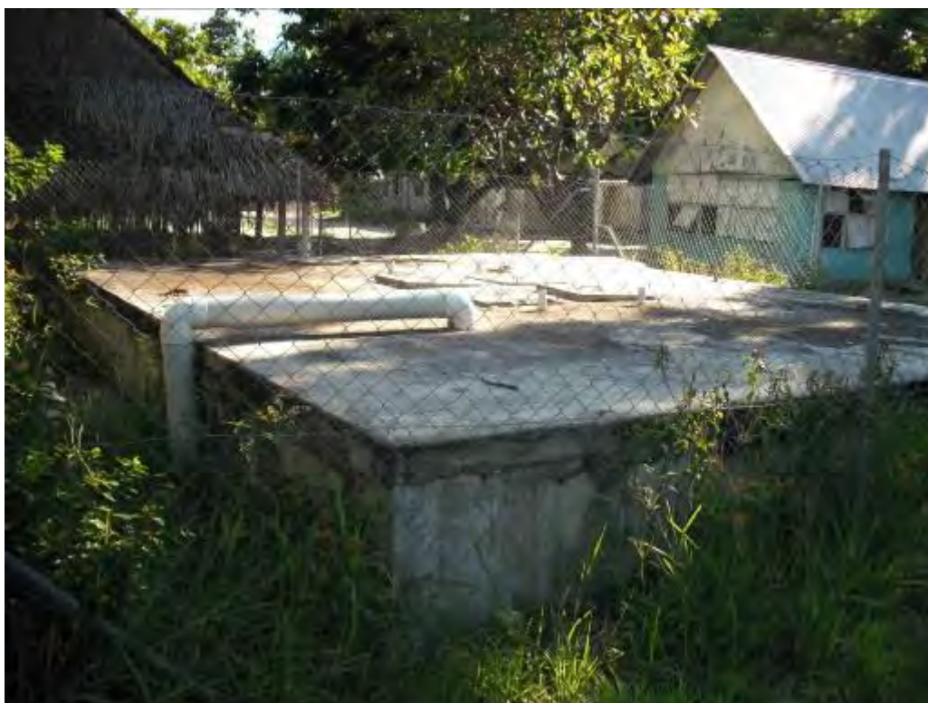
A1.3.7 Large semi-submerged reinforced concrete cistern.
