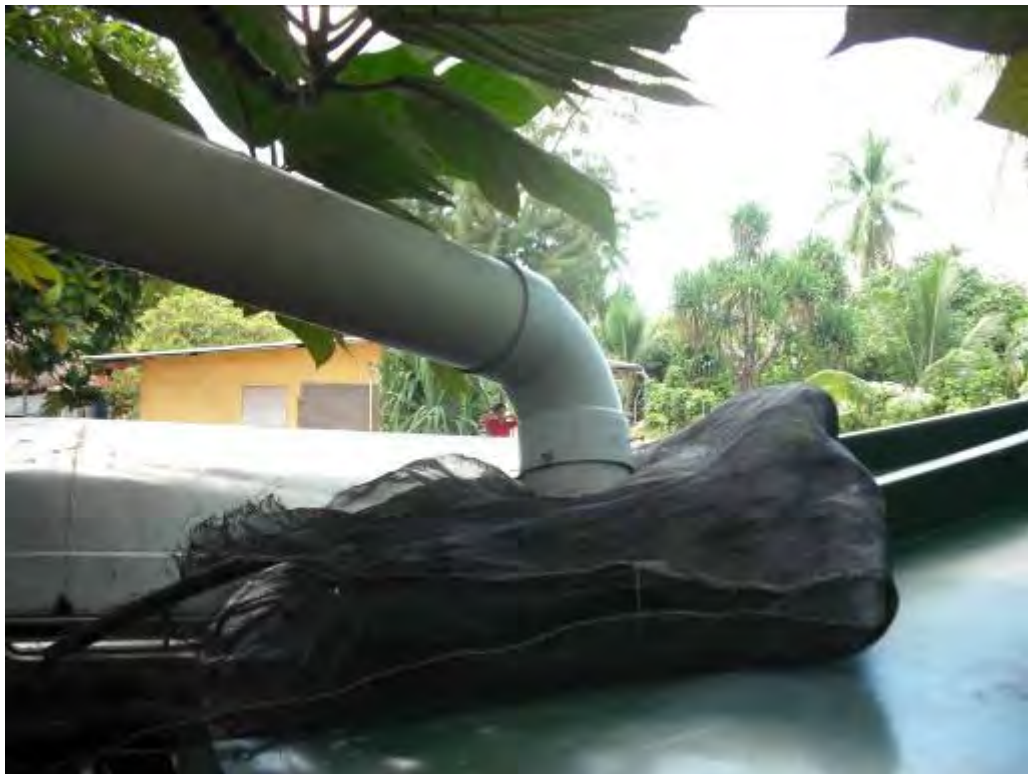
A1.2.3 Makeshift screen using mosquito mesh on tank entry.
