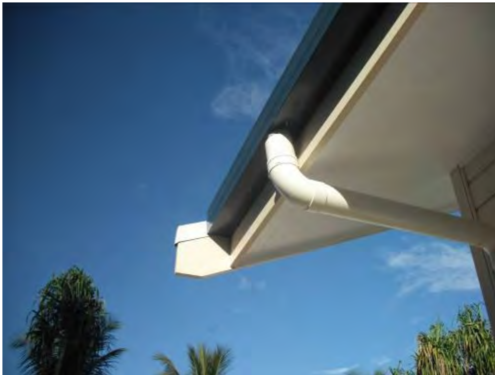
A1.1.15 Good gutter to downpipe connection using a gutter outlet.
