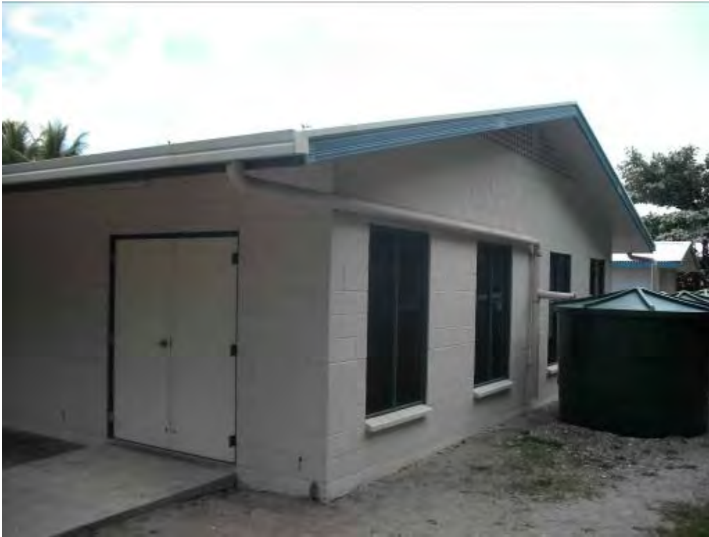
A1.2.1 Simple downpipe first flush device to divert a small quantity of water. Manually operated.
