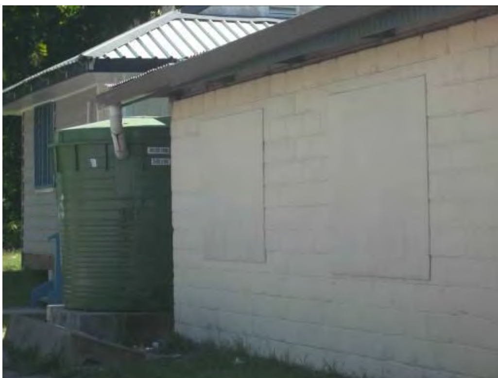
A1.1.13 Good fall on gutter.
