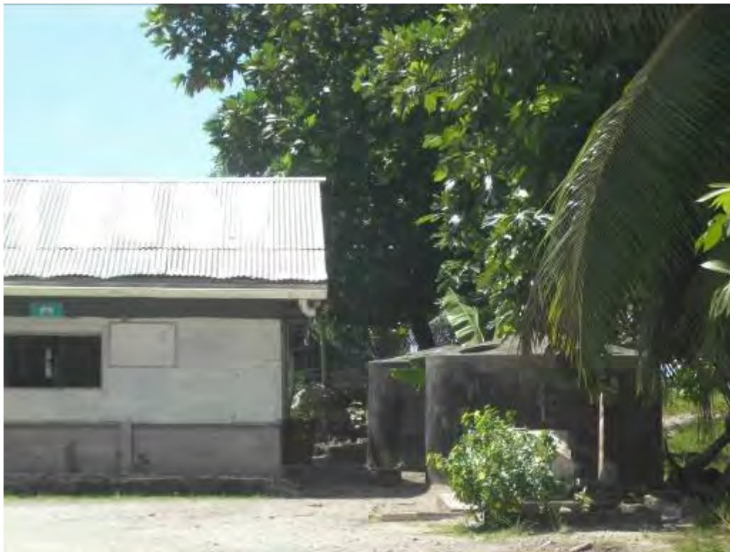
A1.3.3 Unconnected old ferro-cement tanks
